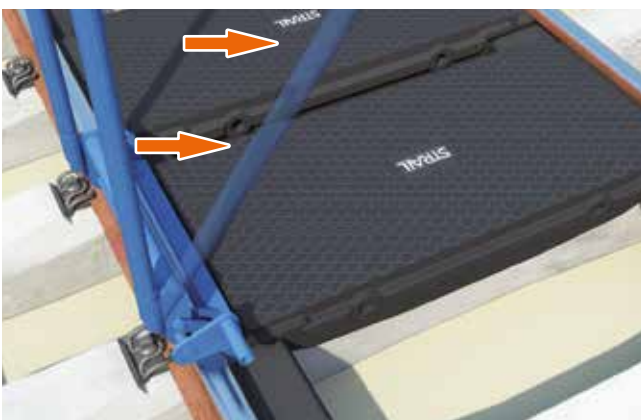
Press the edge of the panel against the installation lever until the lip slides under the rail head.
