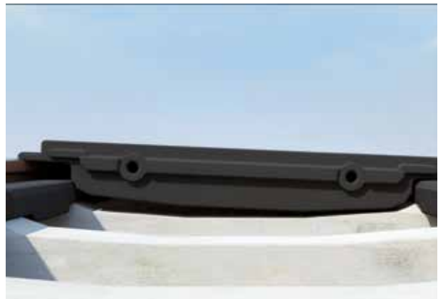
Insert the STRAIL inner panel on one side with its lip under the rail head and grease the lip on the other side with the assembly paste.
