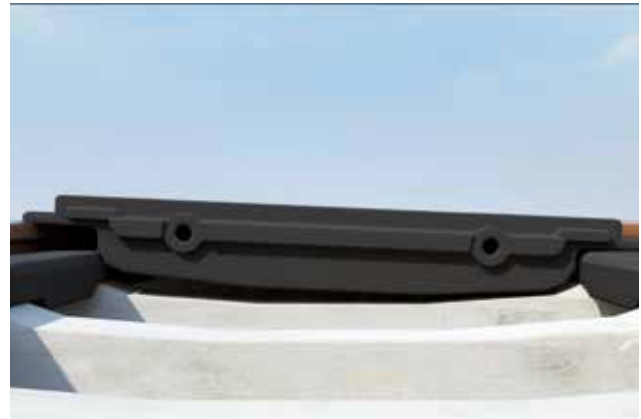
Insert the STRAIL inner panel on one side with its lip under the rail head and grease the lip on the other side with the assembly paste.
