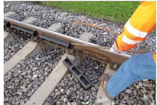
The **STRAILastic\_A synth** damper can be easily removed by use of a standard commercial crowbar.
