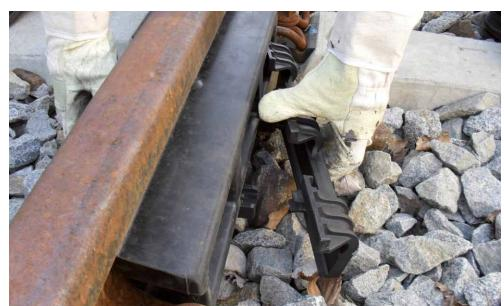
Using the **STRAILastic\_A synth** installation tool (incl. special attachable **STRAILastic\_A synth** attachment) the **STRAILastic\_A synth** clamps are pressed into the sleeper bay, so that the clamps snap into their final position.
