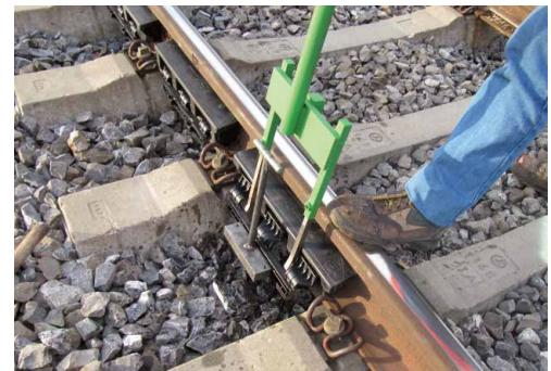
Drive the **STRAILastic\_A synth** expanding mandrel into the respective holes of the fixing clamp with hard blows of the hammer.
